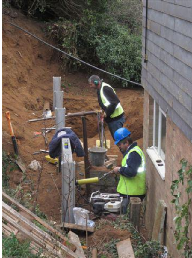
Builders install the new retaining wall
